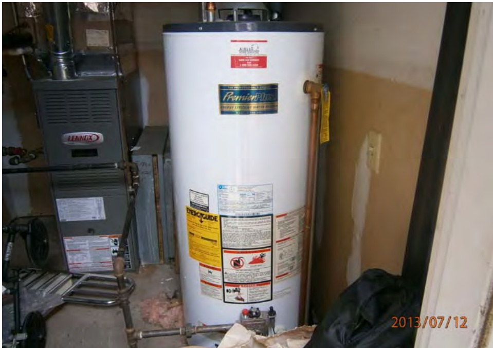
33. Typical unit gas DHW tank
