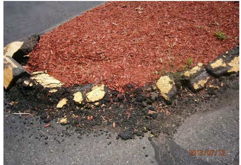
2. Asphalt curbs; damaged
