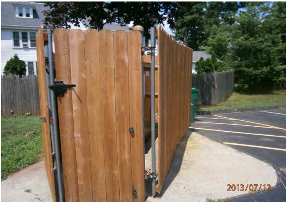
7. Wood plank dumpster enclosure
