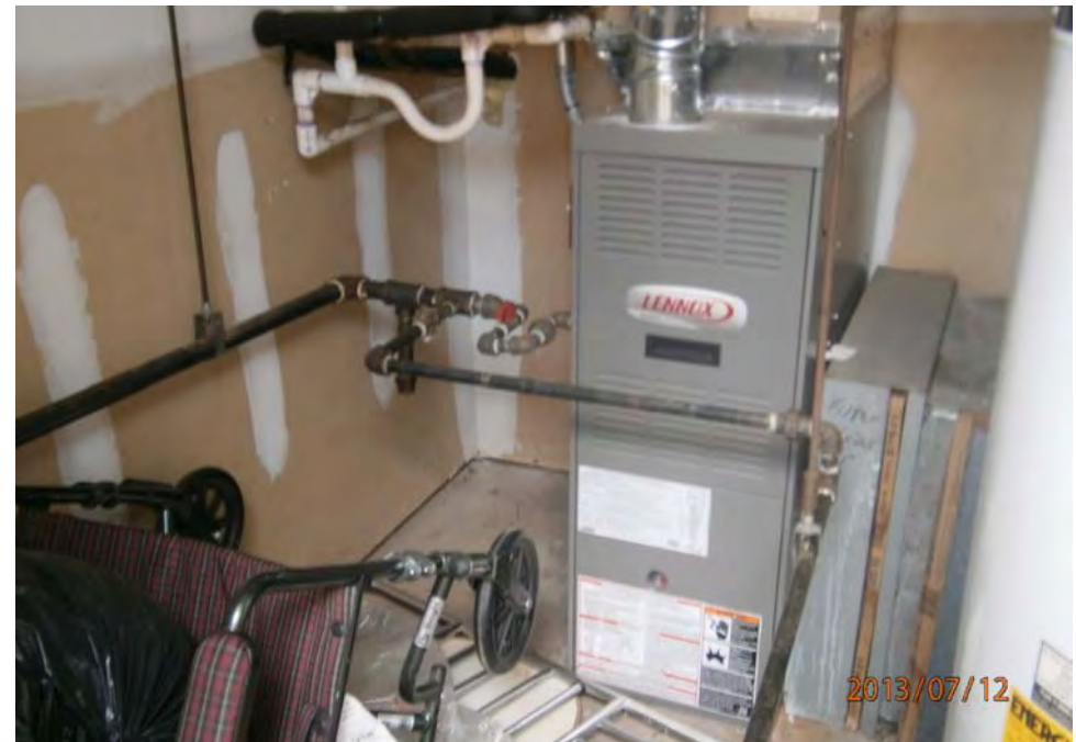
32. Typical unit gas furnace
