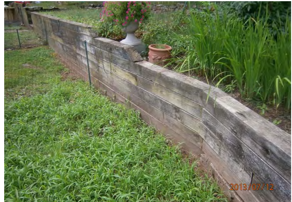
10. Wood retaining wall
